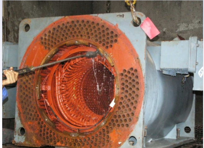
Overhaul of Generators/Motors
